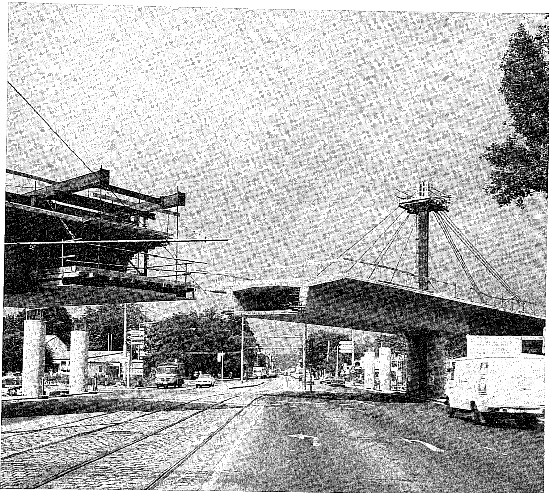
Figure 1.1 - Post-Tensioned Segmental Box Girder Bridge in Construction (From Dywidag Catalog)
